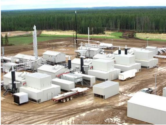
The installation was professional and time-efficient, allowing for minimal interference with the site's normal operation. On each of the five compressor units Noise Solutions installed Acoustical Compressor Buildings, Induced Draft Acoustical Building Ventilation Inlets and Fan Forced Acoustical Building Ventilation Outlets, ensuring superior cooling performance and noise attenuation. For each of the coolers,
