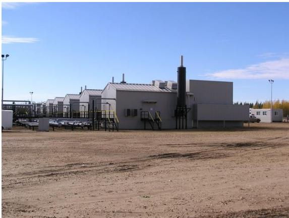
Horizontal Inlet and Outlet Silencers proved to be more than efficient at diminishing the excess cooler noise. For the two additional coolers, Inlet and Outlet Silencers were also used. This combination of noise reduction equipment and design customizations achieved outstanding results.
