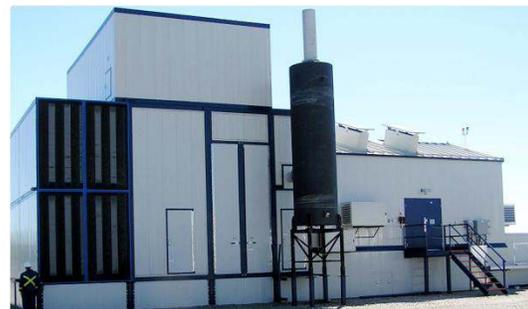
The compressor engine, a Waukesha L5794LT at 1,445 HP, was also equipped with customized Noise Suppression Equipment. This included a full Zeron® Engine Exhaust Silencer package, Induced Draft Acoustical Building Inlet Ventilation and Fan Forced Acoustical Building Outlet Ventilation, as well as an Acoustical Building Enclosure. The combination of this powerful Noise Solutions equipment achieved the goal of zero noise, meeting all regulations.
