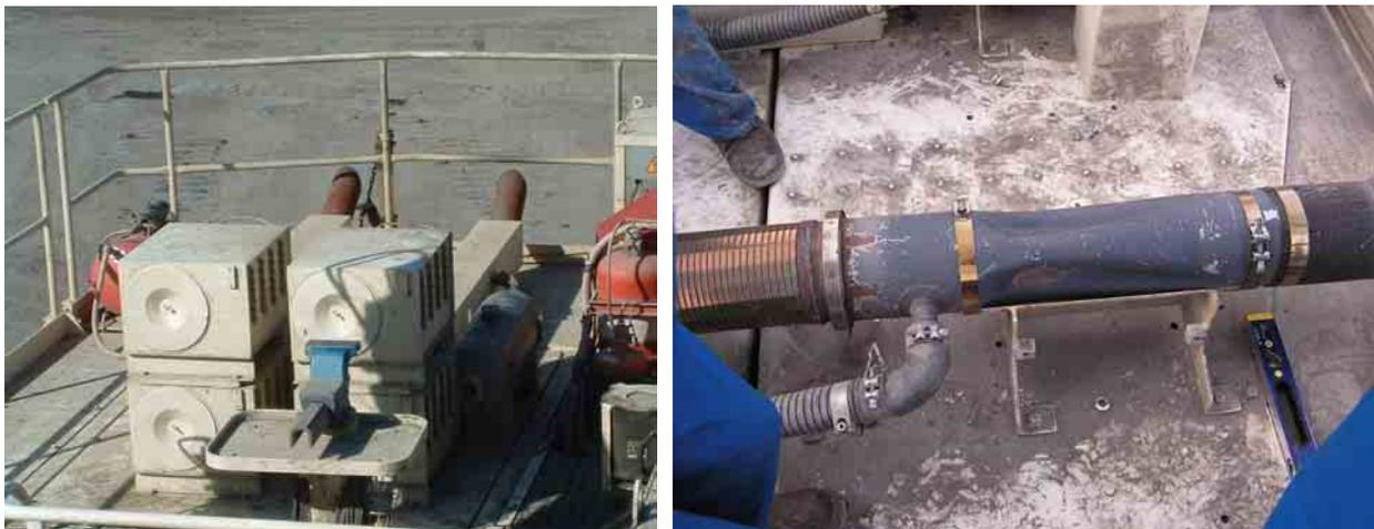
**Figure 4:** Engine air intake filters and exhaust venturis.
